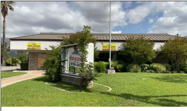
Primary (north) elevation of 101 West Huntington Drive showing monument signage, flag pole, and pathway to front entrance, facing north.
