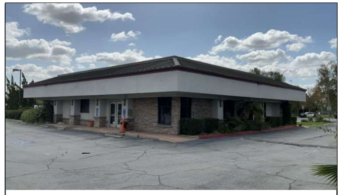
Side (east) and rear (south) elevations of 101 West Huntington Drive, facing southeast.
