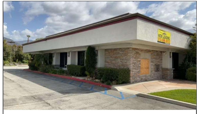
Side (east) and partial primary (north) elevations of 101 West Huntington Drive showing front entrance, facing northeast.
